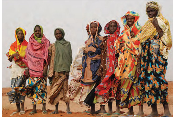
In the Tahoua region of Niger, seven women come together to dig a water catchment structure to help prevent soil erosion. Photo: Michele Egan
