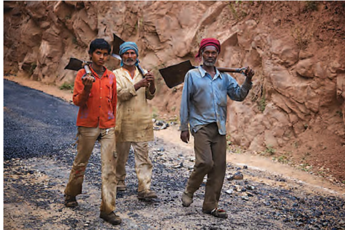
Three construction workers return from a day of work as part of the Rural Roads project to improve access to markets in Rajasthan, India. Photo: Michael Foley
